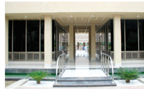
Boys' Hostel- Entrance To T.V. Lounge
