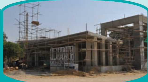
IBA Prayer Hall under construction
